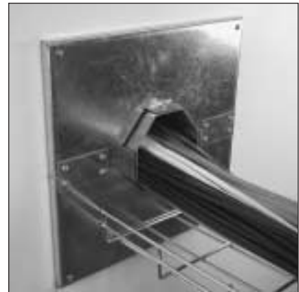
3. Push split conduit into wall.
