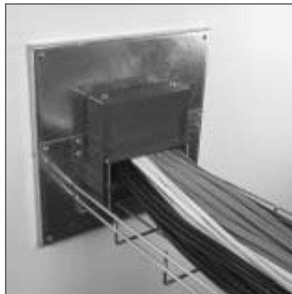
5. Attach FlameStopper box to split conduit.
